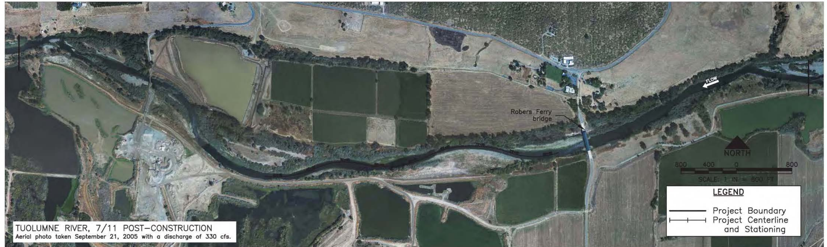
Figure 3-3. 7/11 Reach pre-project (1998), as-built (2002), and post-project (2005) aerial photographs, continued.
